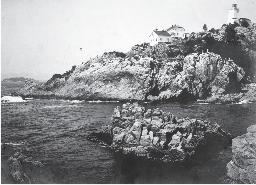
Figure 4. The Cape Beale Lighthouse as seen from the southwest. The rocky waters offshore made this a treacherous coastline. Image P-G04.415 reproduced with permission of the Bamfield Community Museum and Archive.
