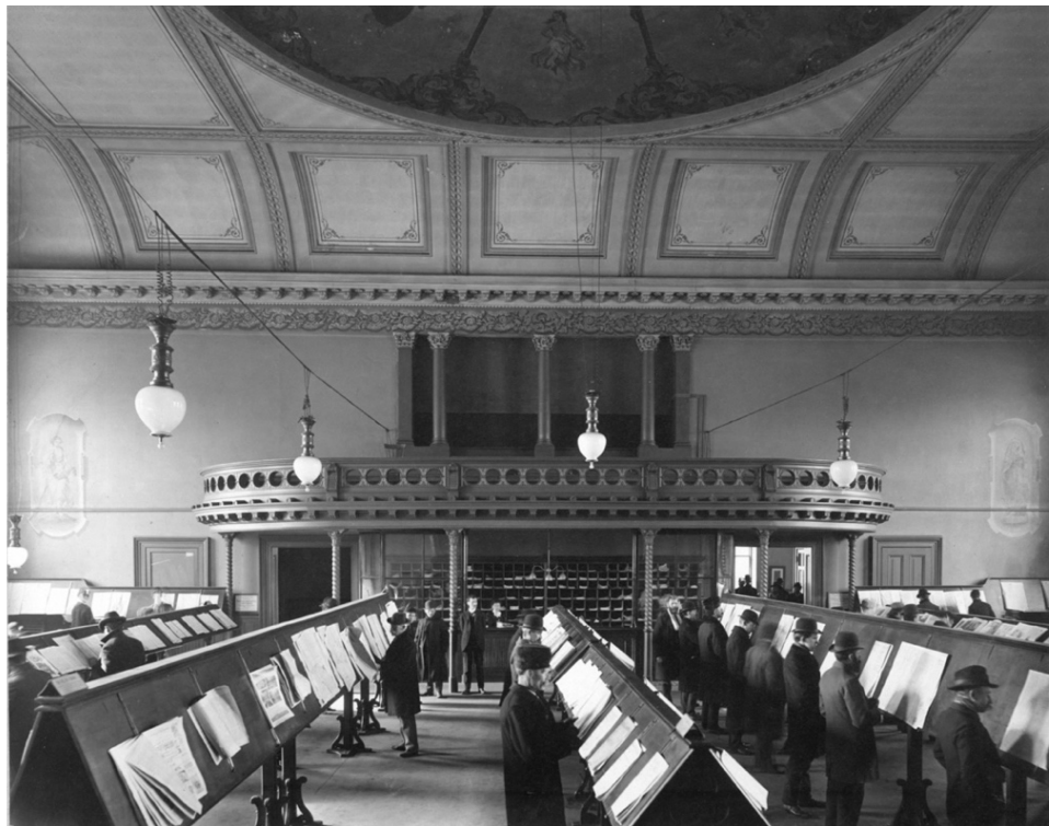
Fig. 2.3 Newspaper room interior, old central library, 1900 19
