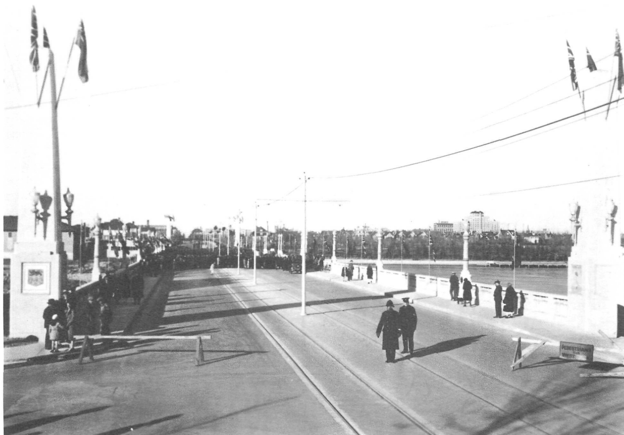
Official opening of the Albert Memorial Bridge, November 1930. This was Regina's first major unemployment relief work project. Saskatchewan Archives Board. R-B1065(1)
